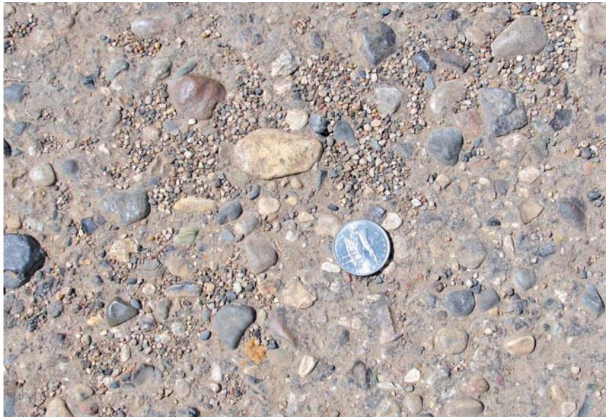
Close-up view of large aggregate used in Otta Seal surfacing.
