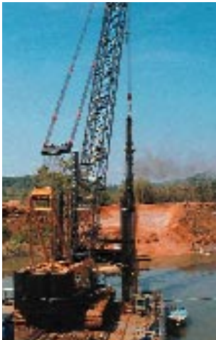
30 inches piles driven with diesel hammer.
