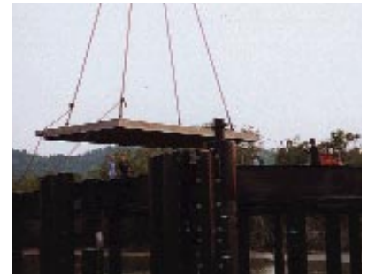
Concrete slabs weight up to 40 tonnes.
