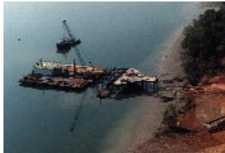
200 tonnes construction barge at work in the Heinze river.
