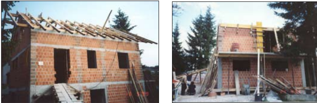
Figure 3: Confined masonry housing during construction in Slovenia (WHE Report 88)
