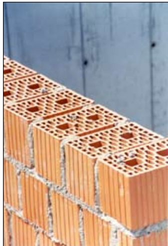
Figure 4: Masonry units used in confined masonry construction (left, Slovenia, WHE Report 88) and a detail of floor construction (right, Serbia and Montenegro, WHE Report 69)
