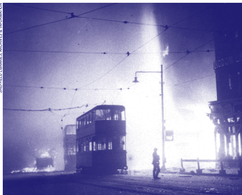
LEFT TO RIGHT: High Street in flames, The Quadrangle in 1944 with air raid precautions in place, Fire fighting.
