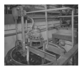
**Fig. 2-21.** Interior view of the Phosgene Production Plant at Edgewood Arsenal, Md. The low level of chemical engineering technology apparent in this World War II– era photograph is relevant to the problem of chemical agent proliferation today. Elaborate, expensive equipment is not required for mass-producing the less-sophisticated chemical agents. Photograph: Chemical and Biological Defense Command Historical Research and Response Team, Aberdeen Proving Ground, Md.
