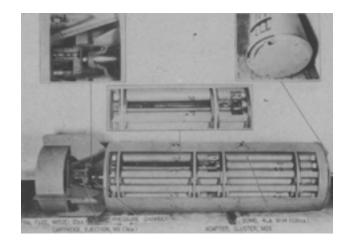
**Fig. 2-47.** The M33 500-lb biological cluster bomb, which held 108 of the M114 bombs. Photograph: Chemical and Biological Defense Command Historical Research and Response Team, Aberdeen Proving Ground, Md.
