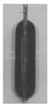
**Fig. 2-10.** Sectionalized view of a Livens projectile. The central tube contains a small explosive charge, which, when detonated by the contact fuze, breaks the shell and aids in the dissemination of the chemical agent. The usual weight of the chemical agent was 30 lb; the shell weighed an additional 30 lb. Photograph: Chemical and Biological Defense Command Historical Research and Response Team, Aberdeen Proving Ground, Md.
