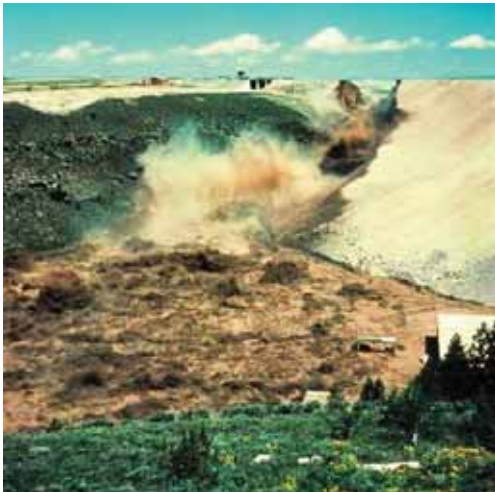
1976 Teton Dam Failure / Source: www.damsafety.org
