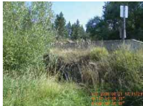
North Viola Bridge in Latah County, before and after mitigation. Note that the small opening, which resulted in backwater flooding, was replaced with a wider span. Funding Source: HMGP, DR-1630.
