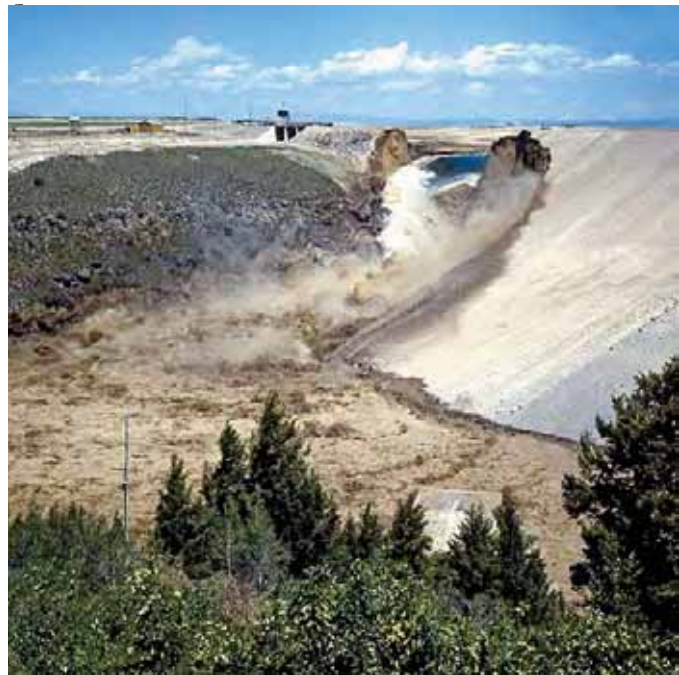
Teton Dam Failure, June 1976. During the first filling of the reservoir, the dam burst when the water was 270ft deep. It drained in less than 6 hours, setting off more than 200 landslides in the canyon below, taking 11 lives, and causing millions of dollars in property damage. / Source: www.damsafety.org
