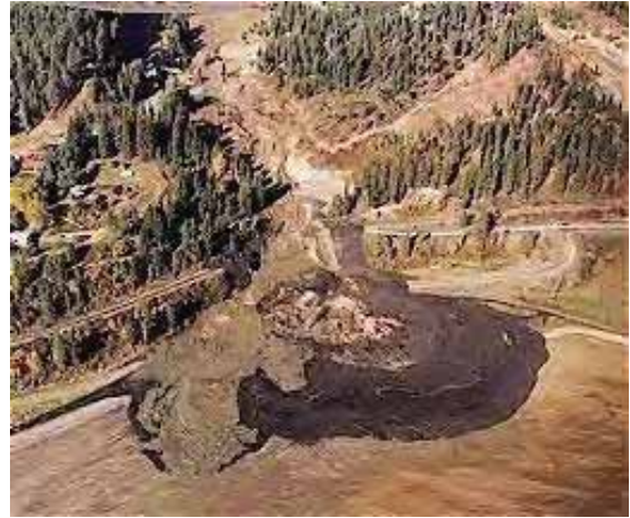
U.S. Highway 95 Bonners Ferry Landslide, 1998 / Source: www.landslidetechnology.com/landslides/bonners_ferry.htm
