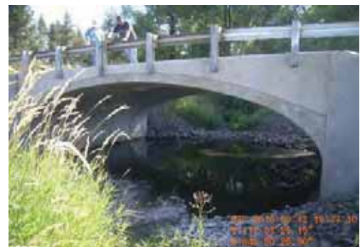
North Viola Bridge in Latah County, before and after mitigation. Note that the small opening, which resulted in backwater flooding, was replaced with a wider span. Funding Source: HMGP, DR-1630.
