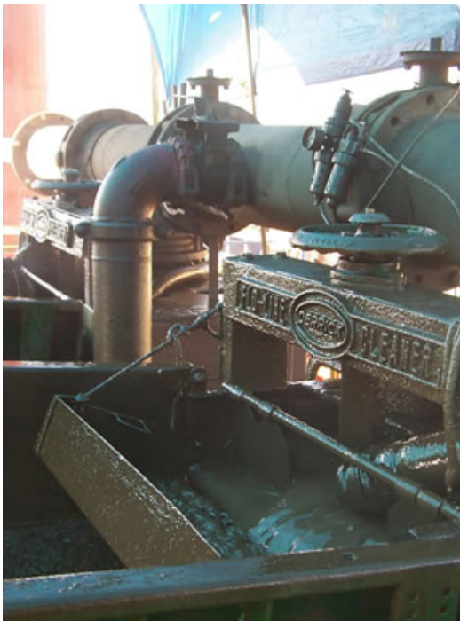
Figure 12: Mud returns at header box
