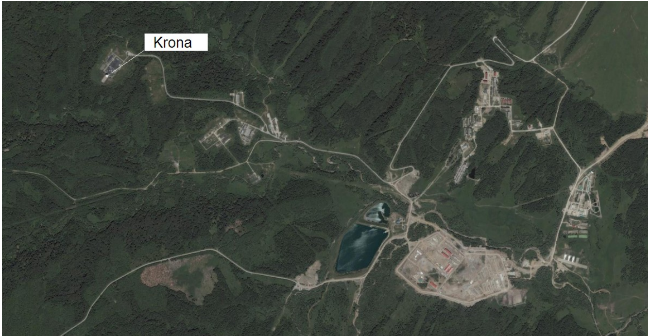
Overview of Krona radar site. Functions of other areas are unknown.
