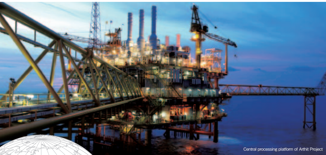
Central processing platform of Arthit Project
