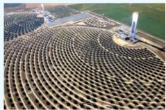
A heliostat field, comprising flat mirrors which track the sun, concentrates the solar radiation on a receiver located on the upper part of a tall tower. Heat is transferred to a fluid (water or molten salts) generating steam that drives a turbine.
