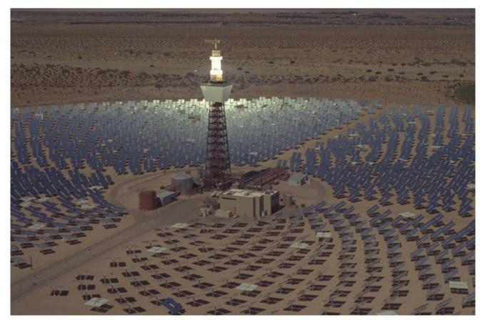
Solar Two in operation at Daggett, California, 1999<sup>2</sup>. Molten salt tanks are the silver pair at base of tower.
