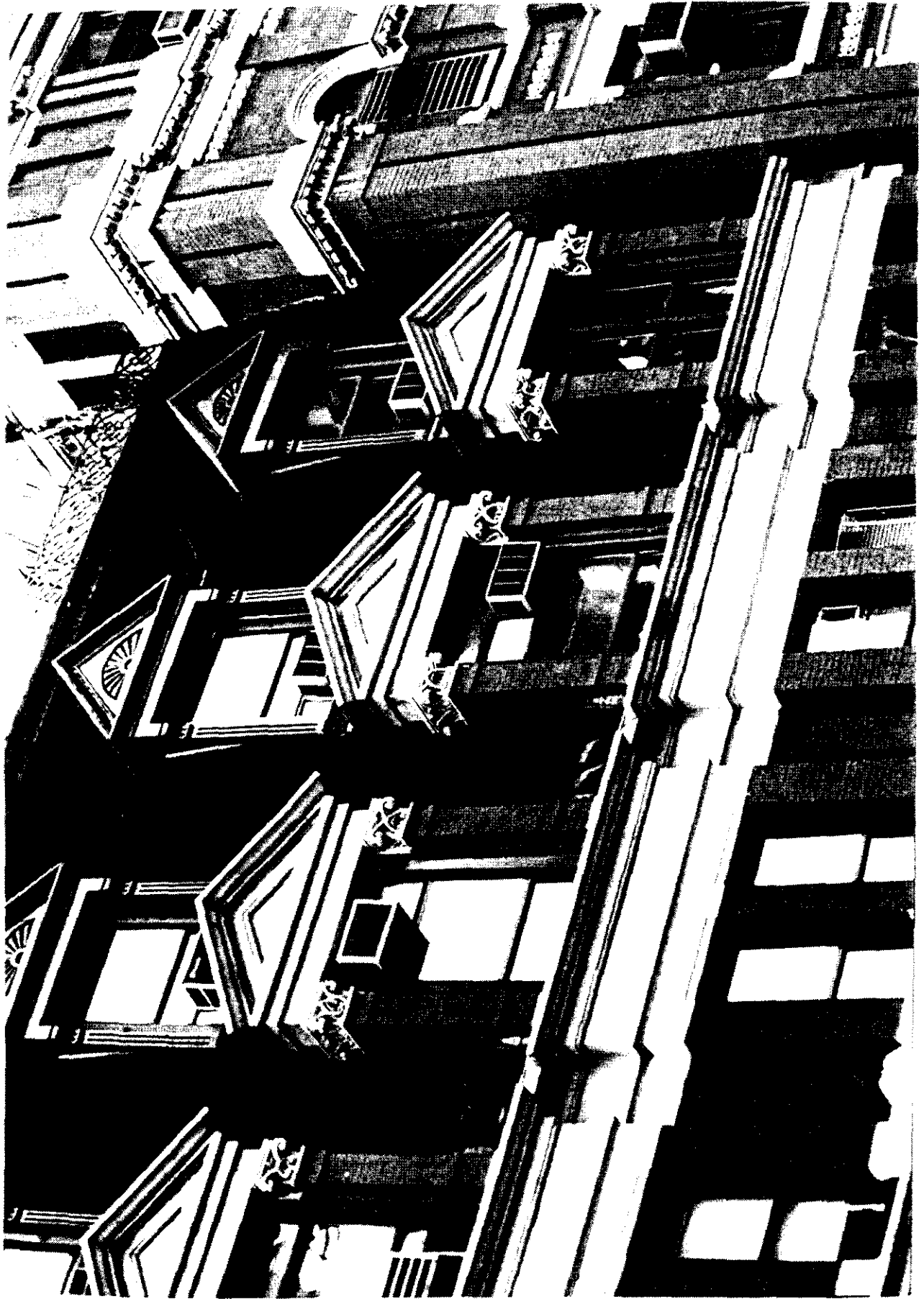
Temple Court Building, Roof Detail Photo: ARCHITECTURE + furniture
