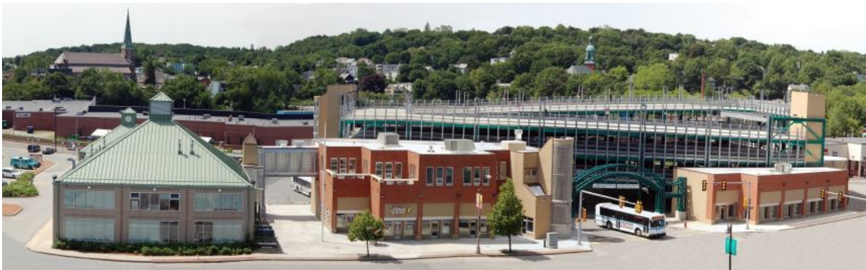
A bus exits the recently-completed Fitchburg Intermodal Center. New retail space can be seen in the storefronts on either side, with the multi-story garage in the background.
