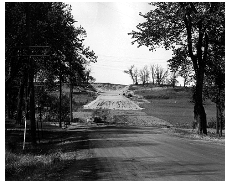
CWA road work
