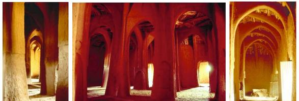
Figure 9: Hypostyle pillars and bent-wood and plastered arches of Yaama Mosque (from http://archnet.org/library/images/one-image.jsp?location\_id=1914&image\_id=13704).
