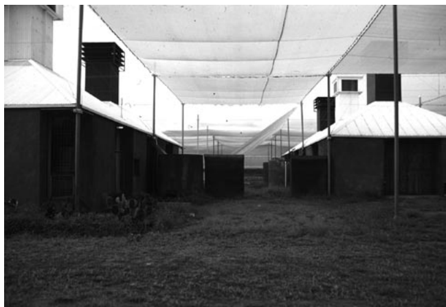
Figure 41: Larado Demonstration Blueprint Farm, Larado Texas. The Center for Maximum Potential Building Systems, Austin, Texas- Pliny Fisk III. 1991.
