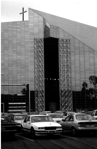
Figure 8 (left): Crystal Cathedral. Exterior view showing 90 foot tall pulpit door open for services.
