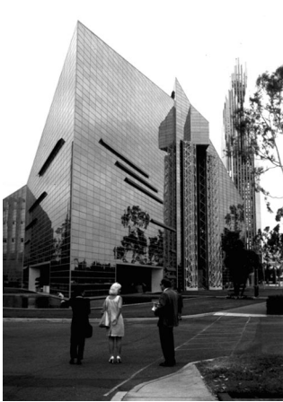
Figure 4: The Crystal Cathedral, Garden Grove, California. Philip Johnson & John Burgee, Architects, 1980.
