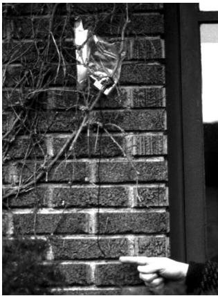
Figure 59 Outdoor air temperature was measured along the north wall during winter and in shade under an eave on the south wall during summer. The HOBO datalogger was placed in a plastic bag, taped shut with duct tape. While the north side sensor location pictured at left was well shielded from solar radiation, the proximity to the wall increased the air temperature reading by roughly 1°F during winter.
