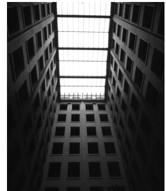
Figure 33: Light court as renovated into an atrium, the Wainwright Building. (Now the Wainwright State Office Complex. Renovation and addition by Mitchell/ Giurgola, Architects in association with Hastings & Chivetta Architects, 1981.)
