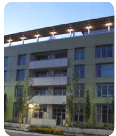
Well designed exterior lighting complements the building design, increases neighbourhood safety and can transform the evening streetscape.
