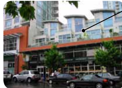
Low rise forms with varying roof heights and changes in plane contribute to the streetscape.
