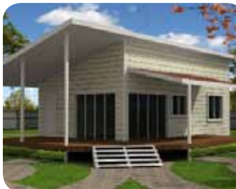
Well designed, contemporary forms including strong, simple roof shapes, large areas of glazing, deck and patio spaces that extend interiors, and simple building forms can be appropriate options for Coach Houses.
