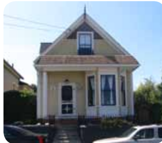
Selected heritage elements including bay windows, simple, steeply pitched roof forms and painted wood cladding are appropriate for heritage style Coach House designs.
