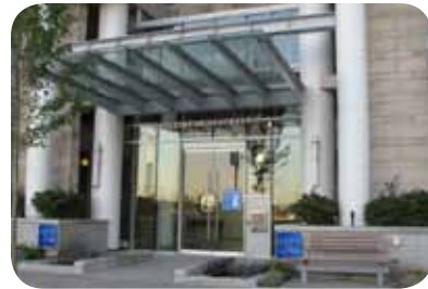
Building entrances should be clearly identified, welcoming, safe, include weather protection and provide architectural interest on the front facade.
