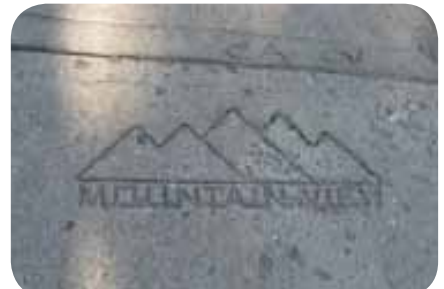
Stamped neighbourhood motifs can be integrated into any new concrete sidewalk surface.
