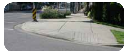
Curb drops are recommended at all intersections.
