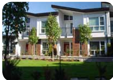
Strong, simple roof shapes and generous glazing proportions provide a modern form to this development. Brick and wood siding refer to traditional residential architecture.
