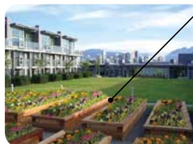
Podium roofs with extensive landscaping slows runoff, reduces heat island effect, provides continuous habitat for birds and increases livability by providing private and common outdoor space.
