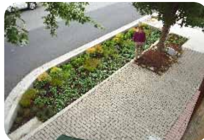
Permeable pavers and boulevard planting increase rainwater permeability.
