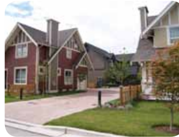
Shared driveways with permeable surfaces
