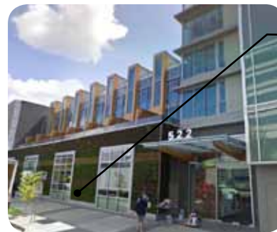
Green walls can reduce the overall temperature of the building, therefore reducing energy consumption, purify rainwater and provide opportunities for community gardens.
