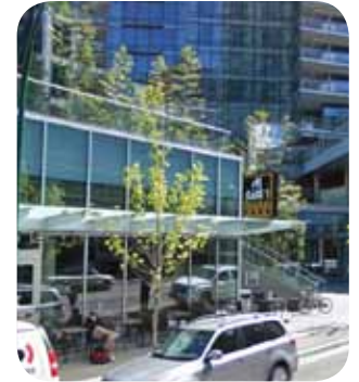
The public realm is emphasized including safe and frequent opportunities to cross the street, enhanced landscaping and places to sit.
