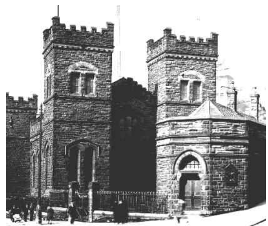
Hydraulic Pumping Station High Street/ Rottenrow Glasgow City Libraries(Mitchell Library)
