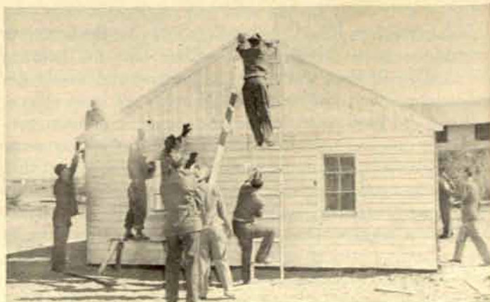
Erecting Gable of Prefabricated House. Two days—2½ Hours later.
