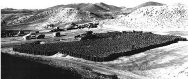
FIG. 2: Contaminated soil and vegetation following the Palomares accident. 1,400 tons of material was packaged in barrels and shipped to the US for disposal. The cleanup and subsequent monitoring cost $120 million. Image from [12]
