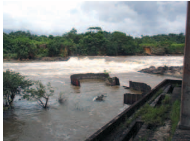
View of St. Paul River from the powerhouse of Mount Coffee hydropower plant in July 2010.
