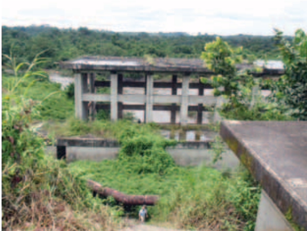
Powerhouse of Mount Coffee Hydropower plant in July 2010.
