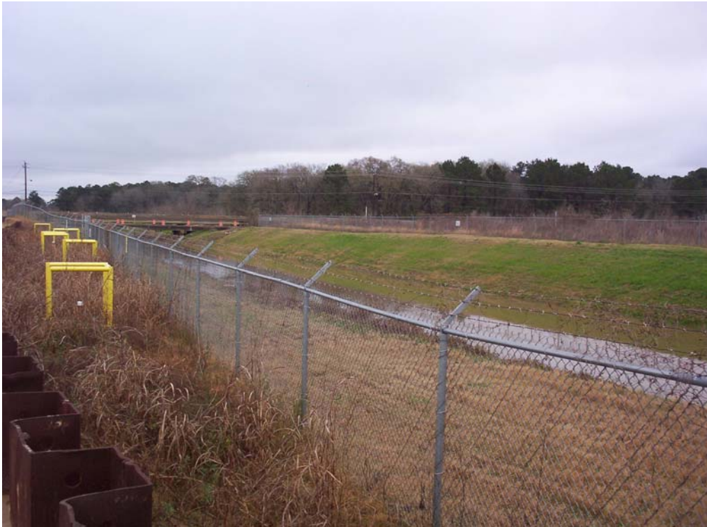
Photo 11. Facing east, looking downstream on Mud Gully. Cofferdam groundwater wells are inside fence on left of photo. Dixie Farm Road bridge is visible in background.
