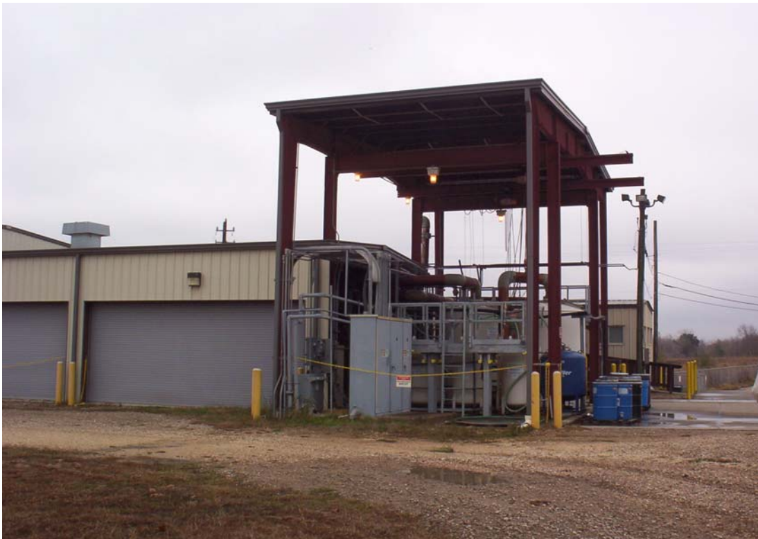
Photo 4. Facing north, southern end of treatment plant.
