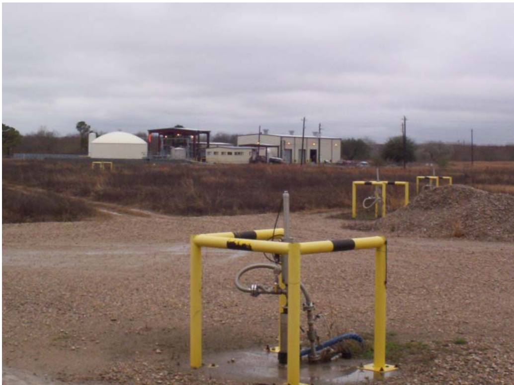
Photo 5. Facing west. DNAPL well B07DW in foreground. Collection tanks, treatment plant and site office in the background.
