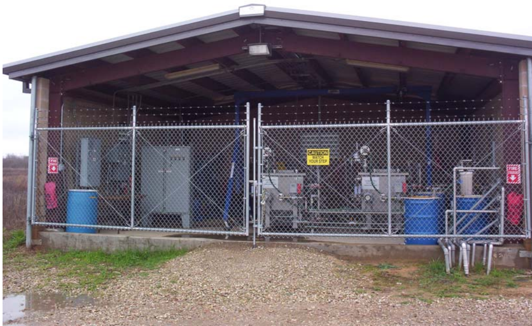
Photo 7. Northwest side of Hub Facility "B".
