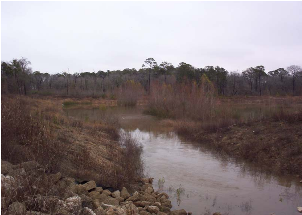
Photo 16. Facing northeast, detention pond created from South Borrow Pit. Picture taken on bank between Mud Gully and pond. Note current from water flowing from Mud Gully into pond following previous night rains.
