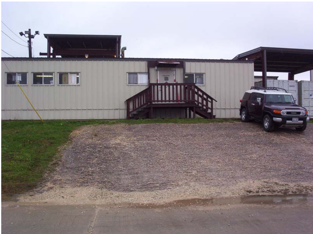
Photo 1. Brio Refining Site Office looking southwest.
