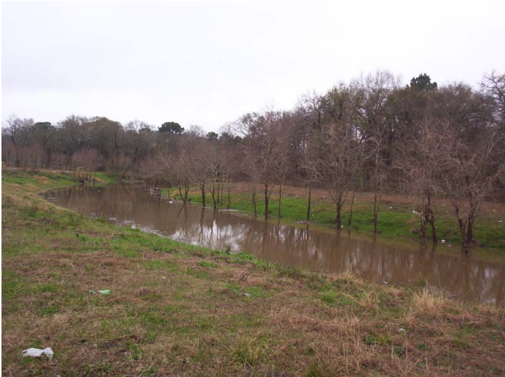
Photo 13. Looking east on Mud Gully, east of South Brio/South Dixie Oil Processor Site.
