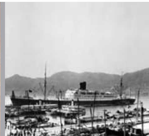
The “Gneisenau” in the port of Hong Kong. The turbine ships were prestigious ambassadors but uneconomical: they carried so much cargo and called at so many ports that they lost the time they gained at sea with their cruising speed of 21 knots.
