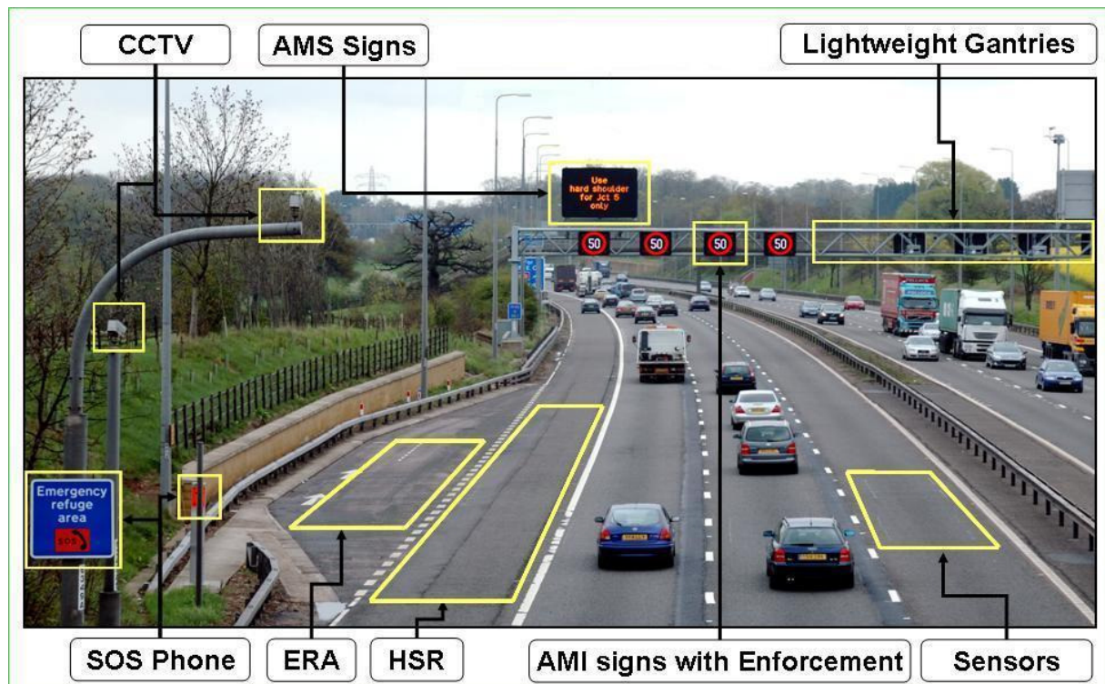
Figure 2.2: Existing and additional technologies required for ATM on the M42.
