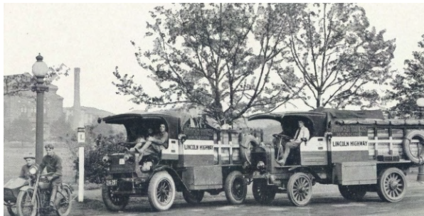
Official Lincoln Highway Association road crews designating the highway alignment in Pennsylvania c.1920, a similar scene would have occurred throughout Nebraska (Photo courtesy of the University of Michigan Lincoln Highway Digital Image Collection)
