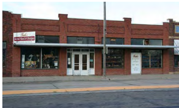
Commercial building in proposed Overton Commercial Historic District
