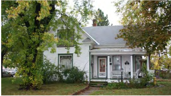
Gable ell in Gothenburg, DS06-135
