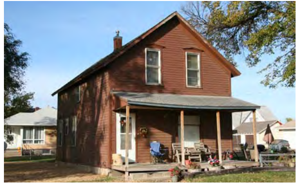
Front gable house in Overton, DS08-030
