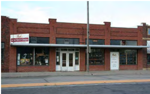
Commercial Building in Overton, DS08-034
