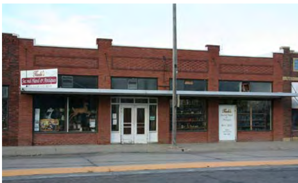
Commercial Building in Overton, DS08-034
