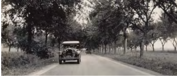
Lincoln Highway Seedling Mile just west of Kearney, c.1915 (photo courtesy of the University of Michigan Lincoln Highway Digital Image Collection)
