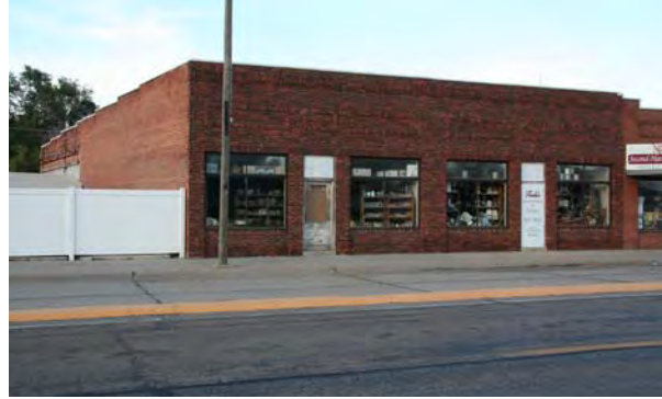
Commercial Building in Overton, DS08-035
