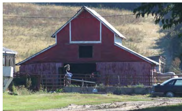
Monitor roof barn near Buffalo, DS00-139
