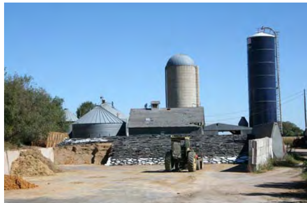
Trench silo near Cozad, DS00-202
