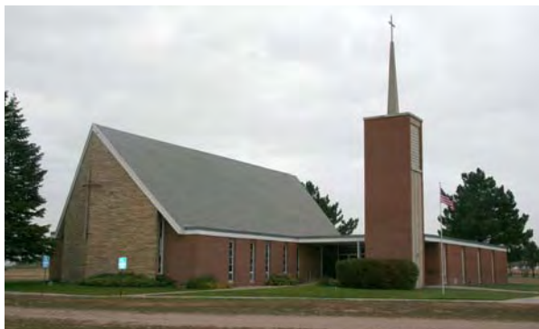
Zion Evangelical Lutheran Church near Gothenburg, DS00-263
