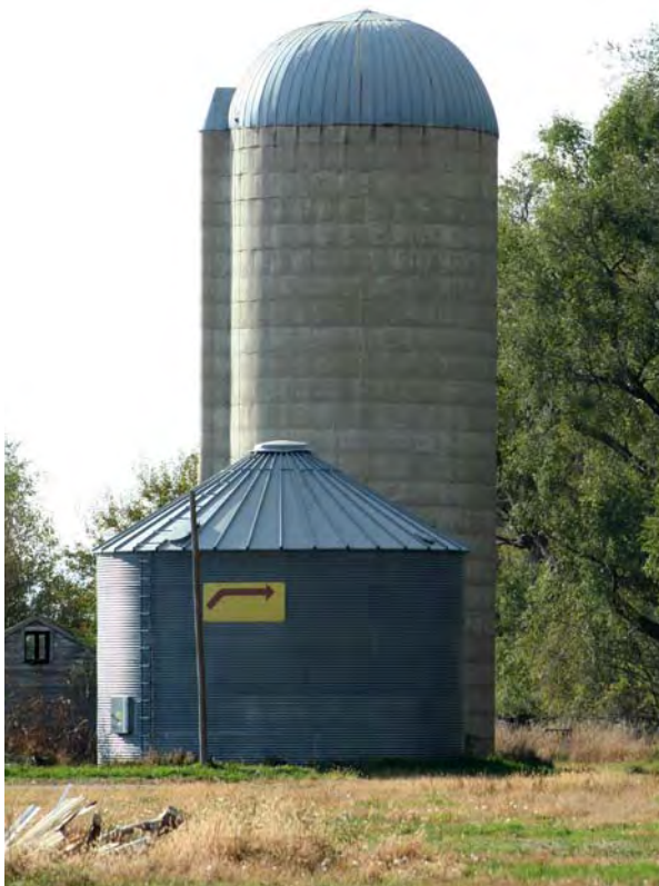
Concrete silo near Gothenburg, DS00-275
