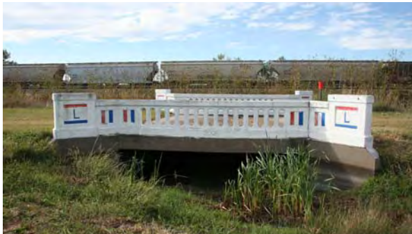
1914 Lincoln Highway Bridge (DS00-018) on original alignment outside Overton
