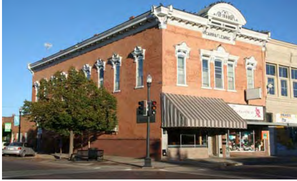
Carr & Fleming Building in Lexington, DS07-006 (in potential historic district)
