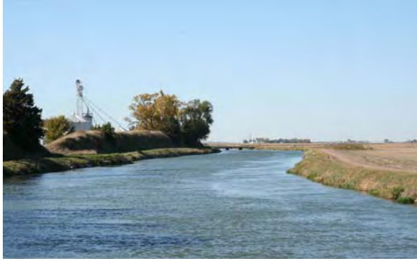
Tri-County Public Power and Irrigation District near Cozad, DS00-019
