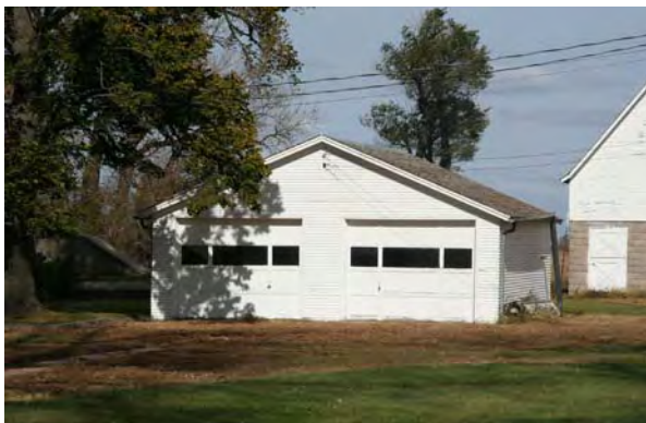
Garage near Willow Island DS00-164
