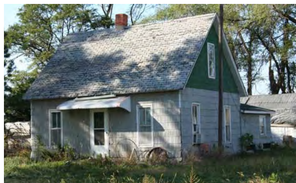
Side gable house in Sumner, DS09-027
