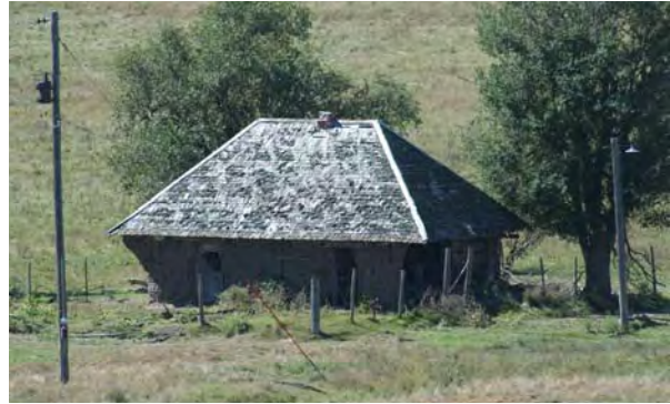
Richardson Sod House near Buffalo, DS00-005
