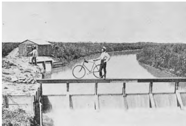
The Farmers and Merchants Canal Company main canal near Lexington, date unknown (photo courtesy of NeSHPO)
