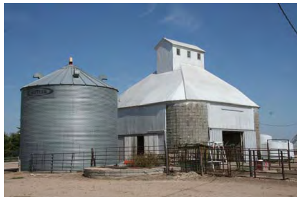
Concrete corn crib with four bins near Eddyville, DS00-070
