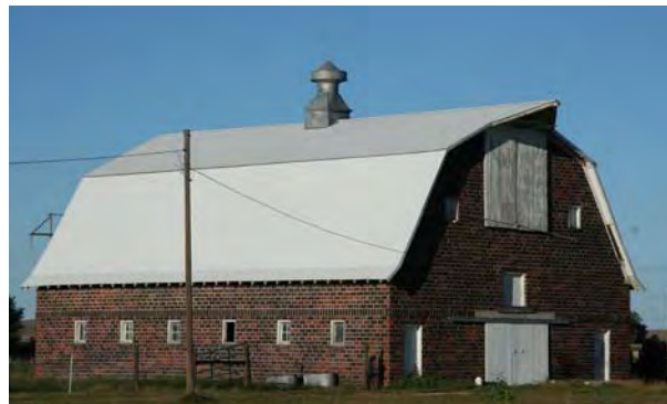
Brick gambrel roof barn near Lexington, DS00-129
