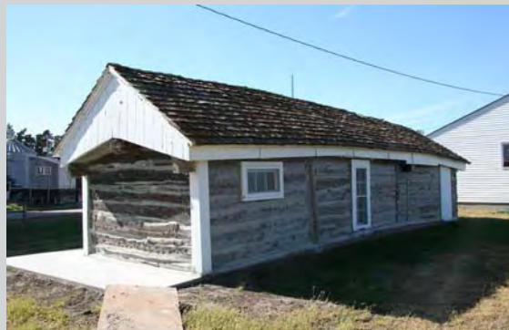
The Pony Express Station (DS00-003) located at Midway Ranch, south of Gothenburg and listed in the National Register
