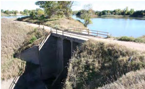
Thirty Mile Canal near Gothenburg, DS00-012
