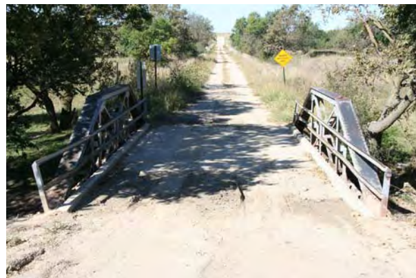
Steel pony truss bridge near Buffalo, DS00-142
