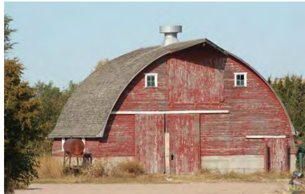
Gothic arch roof barn near Cozad, DS00-223
