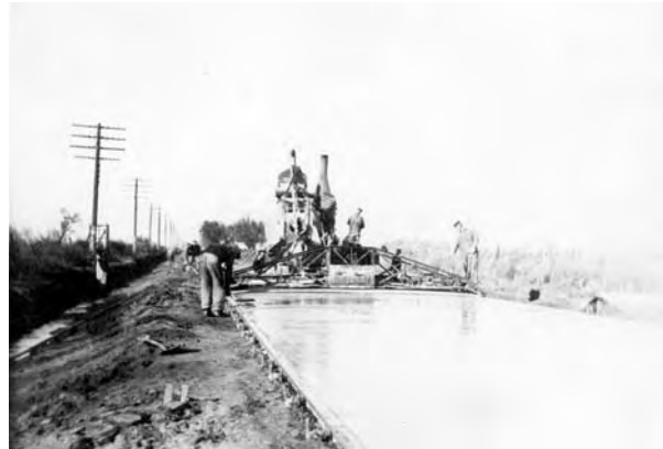
Typical paving operation on U.S. 30 in Dodge County, near Fremont, Nebraska, c.1920 (photo courtesy of NDOR)
