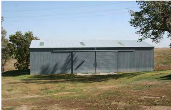
Pole barn near Sumner, DS00-052
