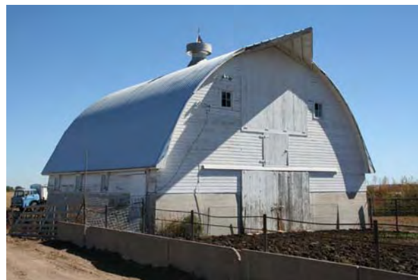
Gothic arch roof barn near Cozad, DS00-201
