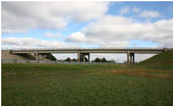
Prestressed Concrete Girder Bridge near Darr, DS00-047
