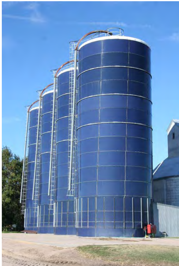
Harvestore silos near Lexington DS00-122
