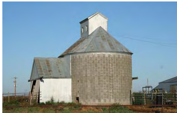
Concrete corn crib with double bin near Lexington, DS00-076
