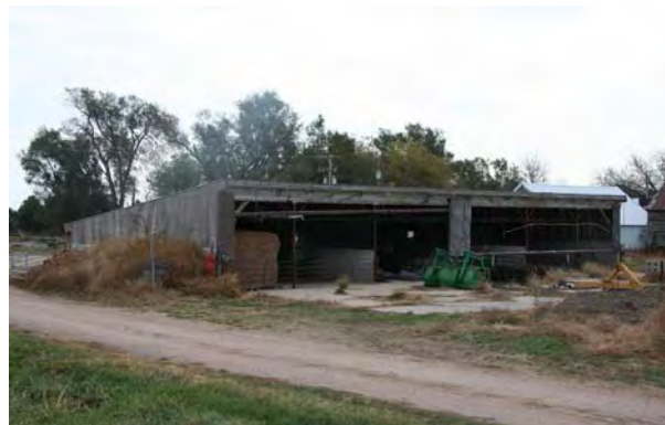
Loafing shed converted to storage building near Gothenburg, DS00-259
