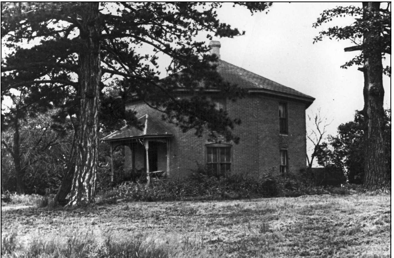
Photo 2. View to the west. Photo by P. Kolberg, 1971, NSHS
