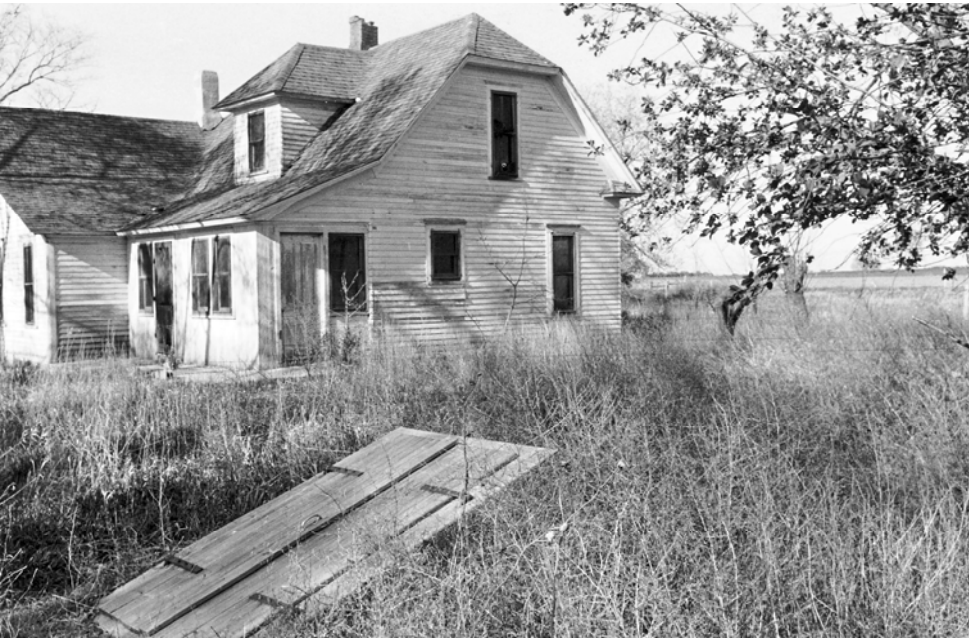
Photo 1– view of house and cellar looking northeast Photo by Dick Spencer, 1978, NSHS (7804/8:5A)
