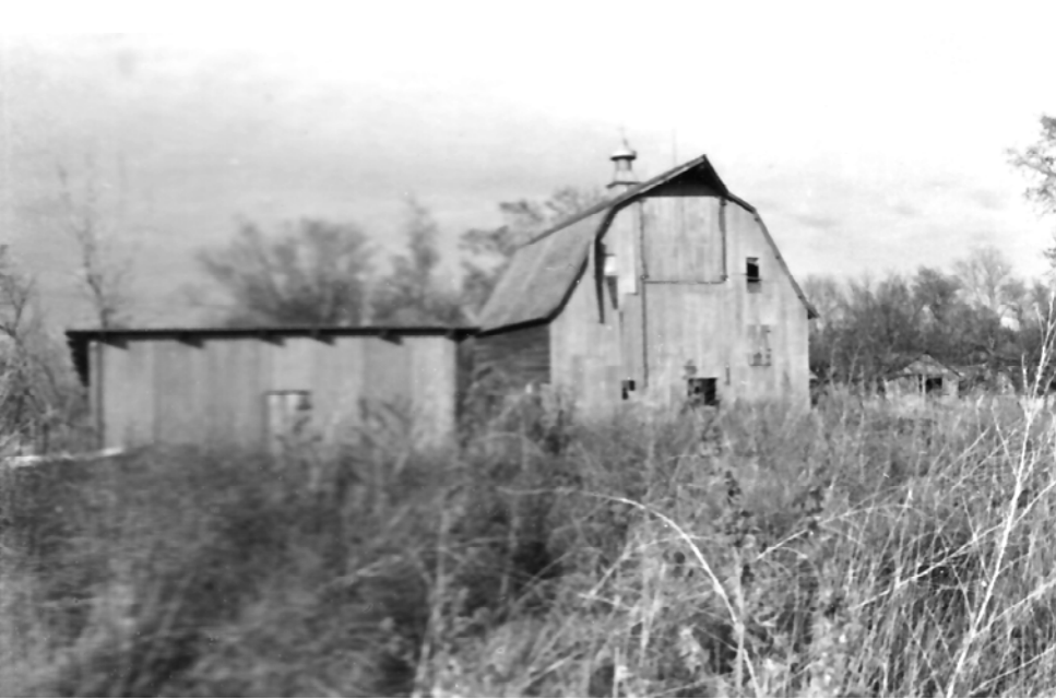
Photo 5– view looking north-northeast showing shed and barn Photo by Dan Kidd, 1978, NSHS (7811/11:8)
