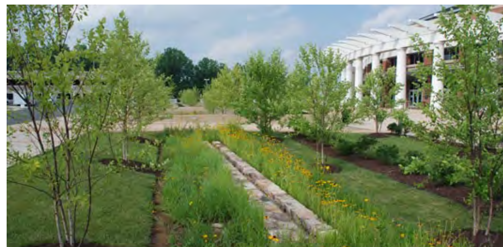
The landscape design of Rain Gardens, Bio-retention Cells, & Stormwater Planters can compliment the geometry and organization of the park. This example employs a clean, architectural design for the stone channel protection that lines the channel bottom.
