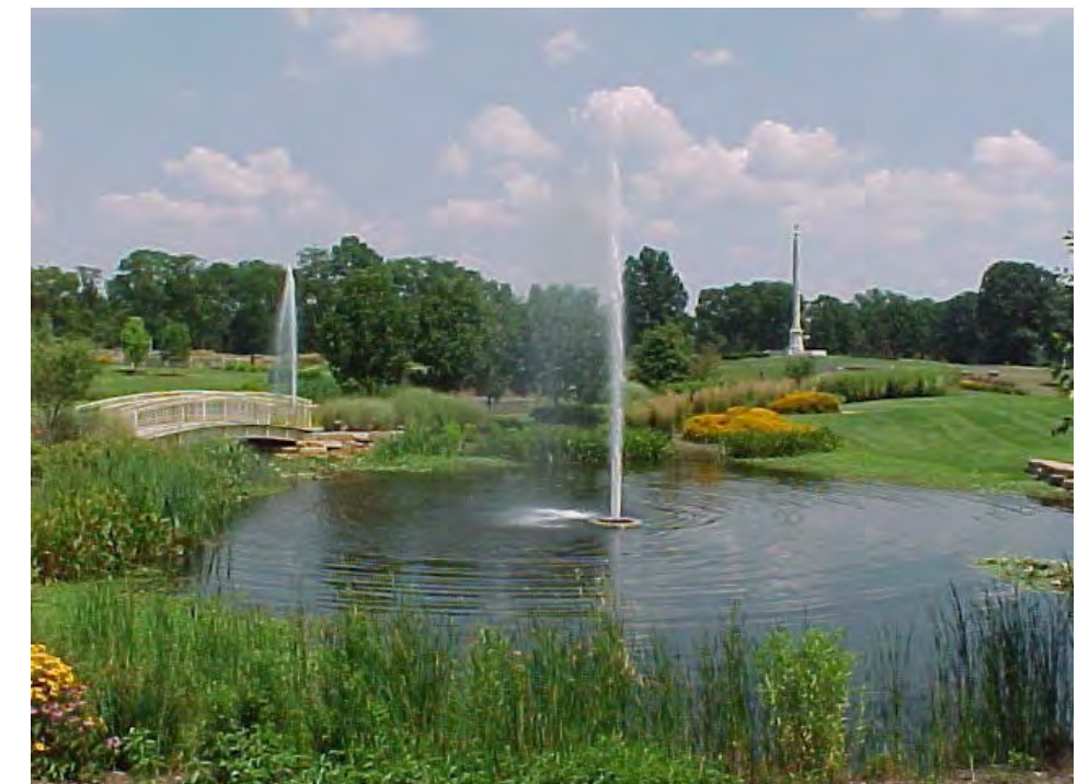
Water Quality & Rainwater Harvesting Ponds such as this example from Gate of Heaven in Montgomery, Ohio provide aesthetic and recreational benefits in addition to providing for the extended detention of and filtering of stormwater flows.
