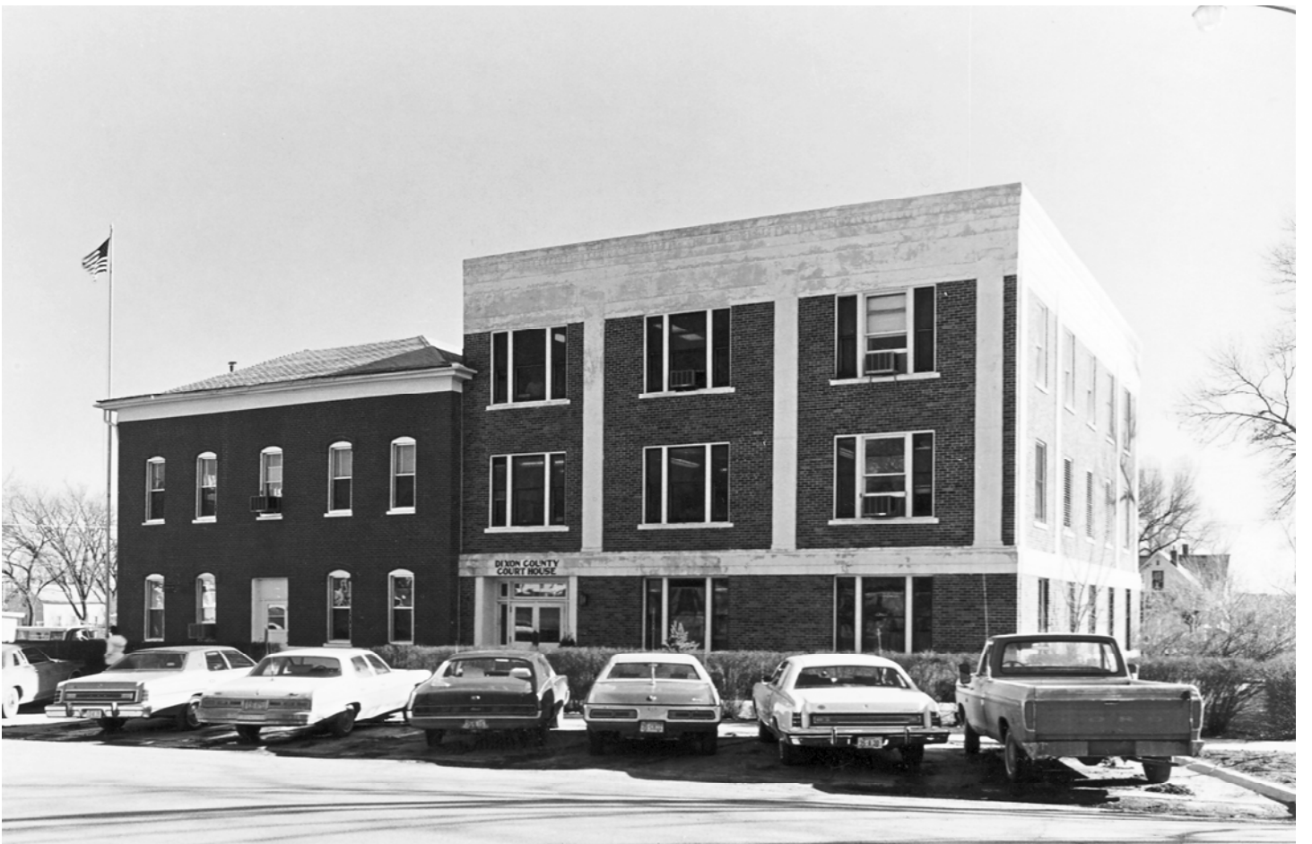
Photo 2—Aspect: north-northwest. Photo by D. Murphy, 1977, NSHS (7703/10:20)
