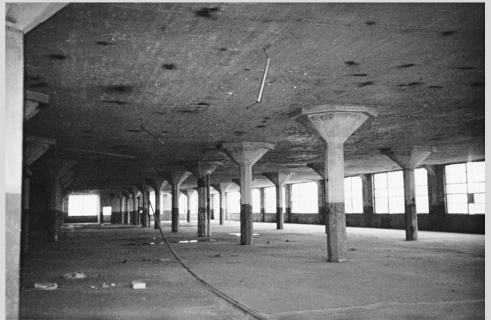
Photo 7 — fifth floor looking southwest
