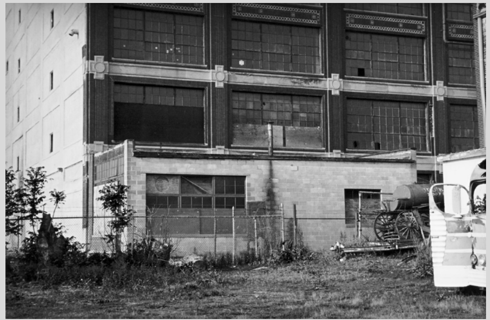
Photo 5 — north façade of north addition
