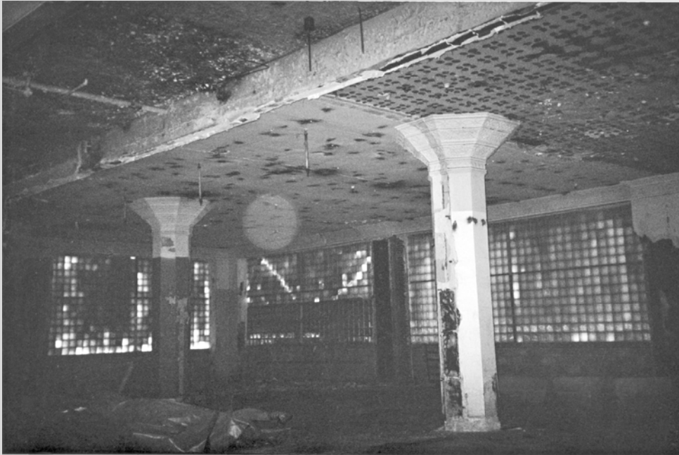
Photo 6 — first floor showroom looking southwest
