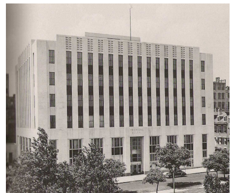
Baltimore Telephone & Telegraph Building (1941) Baltimore, Maryland Source: The Telecommunications History Group, Denver, Colorado
