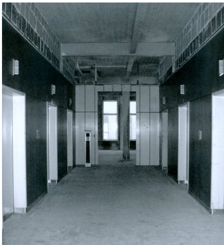
12th floor elevator lobby looking S
