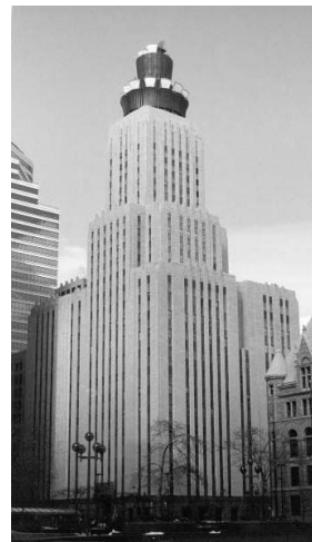
Minnesota Area Headquarters (1931), Minneapolis, Minnesota. Source: Wayne Lorentz/Artefaks Corporation photographer.
