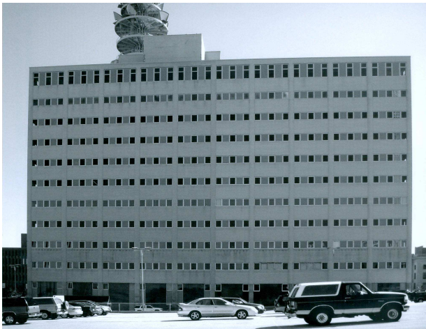
N façade looking S
