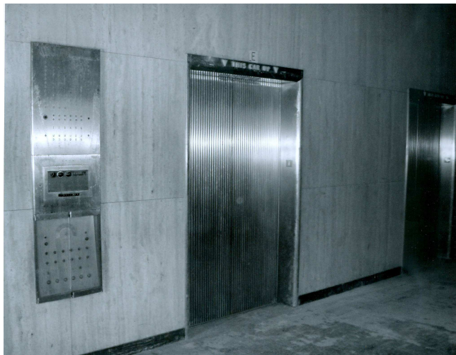
1st floor elevators
