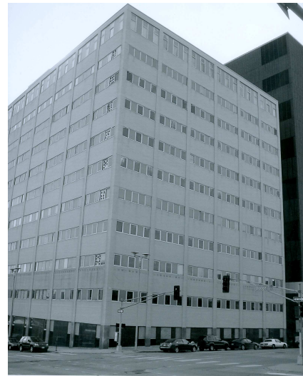
W façade looking SE
