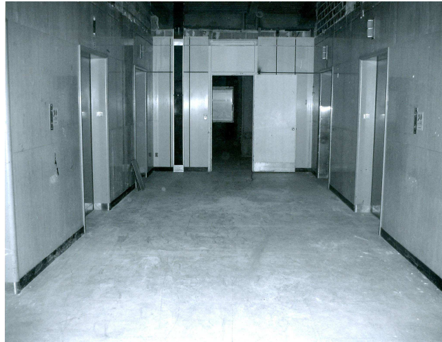
5th floor, elevator lobby looking S
