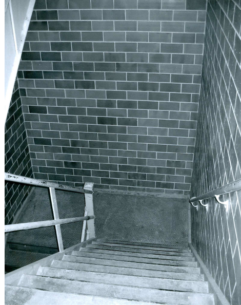
interior stair tower
