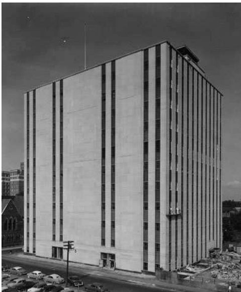
Southern New England Telephone Company Administration Building (1955), New Haven, Connecticut Source: AT&T Archives and History Center, San Antonio, Texas.
