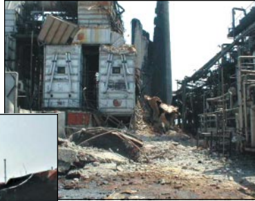
Figure 4. In the photo to the right, a collapsed RC stack is shown. Below, firefighters are cooling burning tanks (source: G. Johnson, EQE International)
