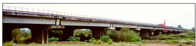
Figure 2. Looking south at the west-bound E80 bridge over the Sakarya River.
