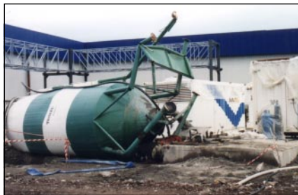
Figure 4. The anchor bolts ruptured and the unbraced support legs buckled, causing this water tank to tip.
