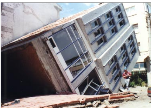
Figure 1. One example of foundation failure.
