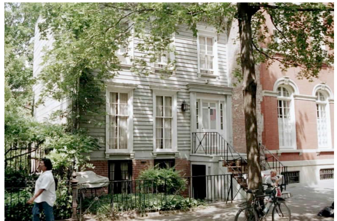
Wood frame building from 1829.
