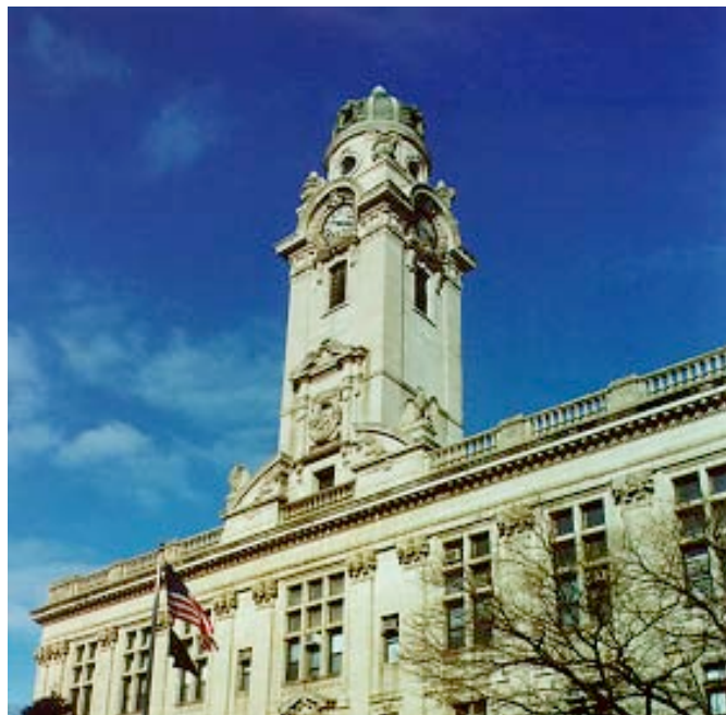
Paterson City Hall , Market St. between Washington and Colt Sts. A three-story gray limestone building with a weathered copper dome surmounting a small tower. Erected in 1894. Rebuilt after a fire in 1902.
