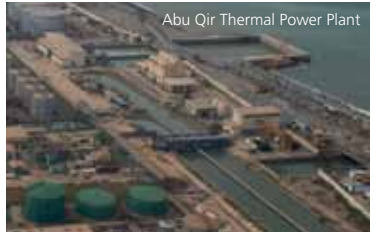
Abu Qir Thermal Power Plant
