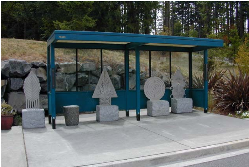
Customized bus shelter: Tree Shelter by Pam Beyette University of Washington/Cascade Community College Bothell Campus
