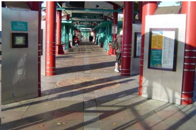
Terrazzo Medallions at Northgate Transit Center Bruch, 1987 Inventory #25a Integrated art enhances site identity, pedestrian experience, connection.
