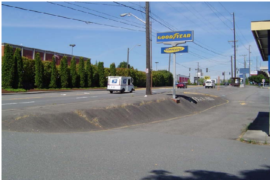
Site of Northgate Civic Center before construction of new park, branch library and community center and construction of 5 th Ave. NE Streetscape Improvements, Phase 1
