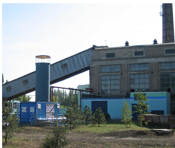
Flare and boiler house, Ukraine
