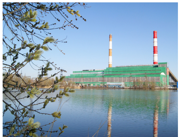
Thermal power plant, Russia
