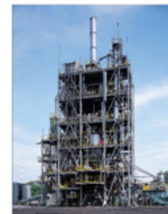
Pilot Plant (20ton/day)
