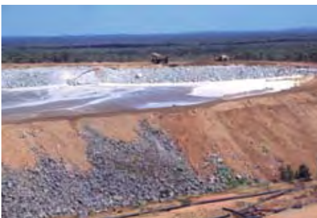
Downstream construction
