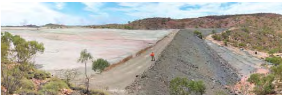
Tailings storage facility downstream containment wall in a dry climatic setting
