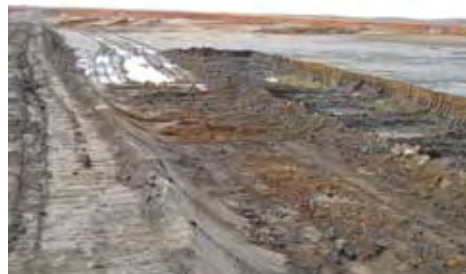
Upstream construction using tailings
