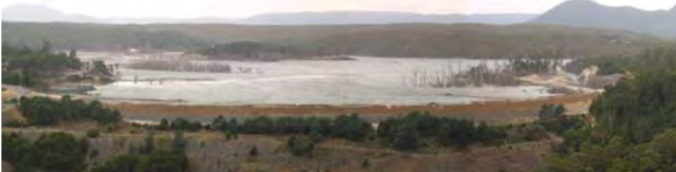
Tailings storage facility downstream containment wall in a wet climatic setting
