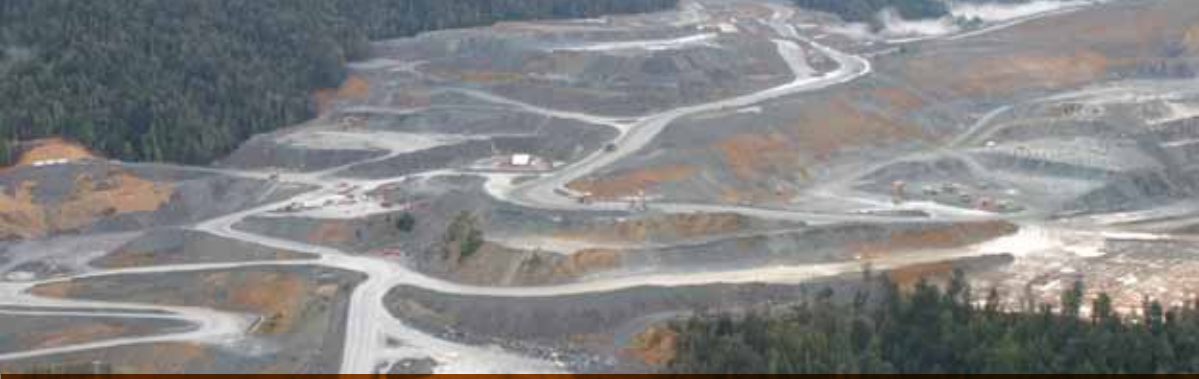
Savage River — helicopter view of Savage River Mine
