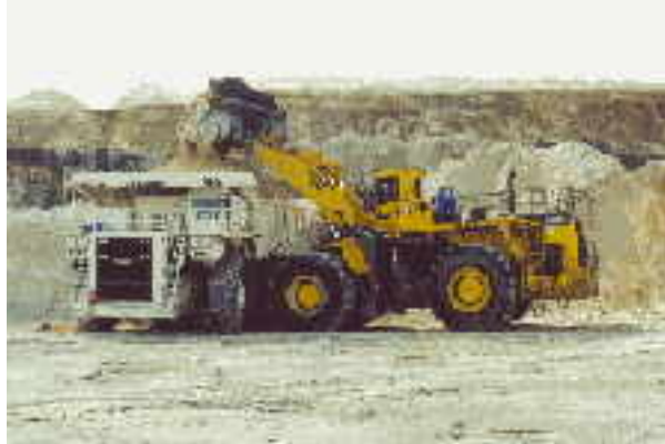
Figure 4.3: Overburden loading by front-end loader Photograph courtesy Griffin Coal
