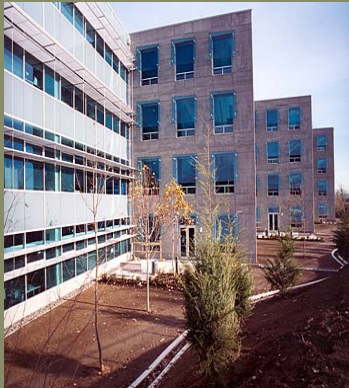
BC GAS BUILDING, SURREY
