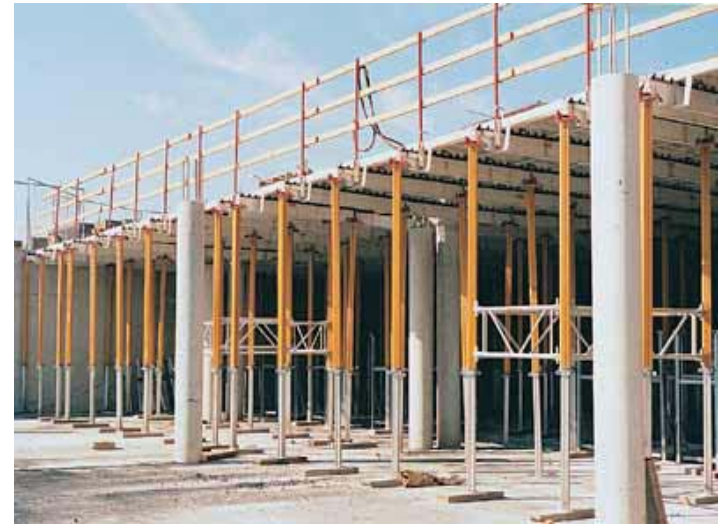
PROPRIETARY FORM SYSTEM
