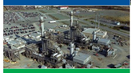
Grandview is an 88 megawatt gas-fired cogeneration power plant that is situated within the Irving Oil Refinery in Saint John, New Brunswick. Under a 20-year tolling arrangement, Irving will provide fuel for the plant and contract for 100 per cent of the plant's heat and electricity output.
