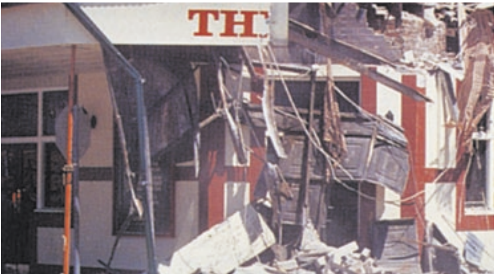
SEVERE DAMAGE TO THE KENT HOTEL, NEWCASTLE, 1989.
