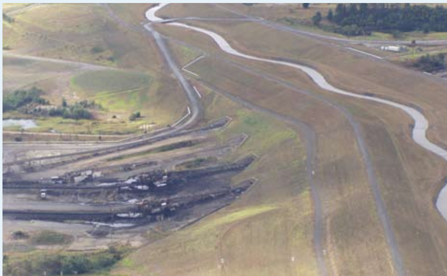
Aerial photo of northern section of Morwell River Diversion at confluence with Latrobe River showing coal supply conveyor tunnels and road ramp/crossing.
