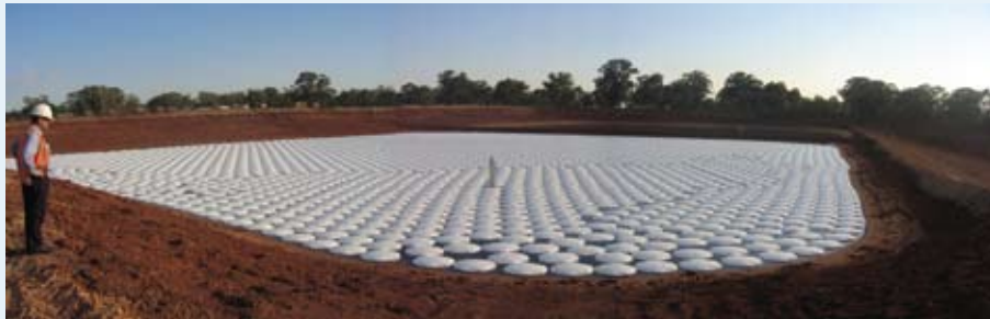
Floating modules on water storage dam at Northparkes mine. Image source: Rio Tinto
