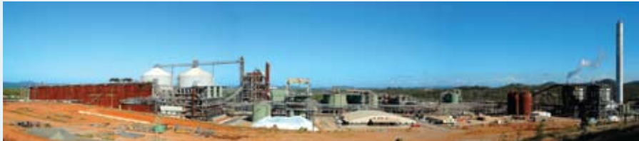
Rio Tinto Aluminium Yarwun alumina refinery. Image Source: Rio Tinto
