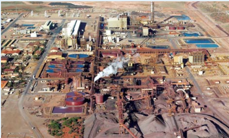
Aerial Photo of Olympic Dam Processing Plant. Image Source: BHP Billiton
