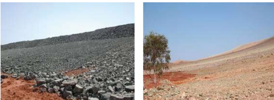
Figure 8. Outer slopes of waste rock dumps: (left) Bi-linear batter slope and (right) continuous concave batter slope.
