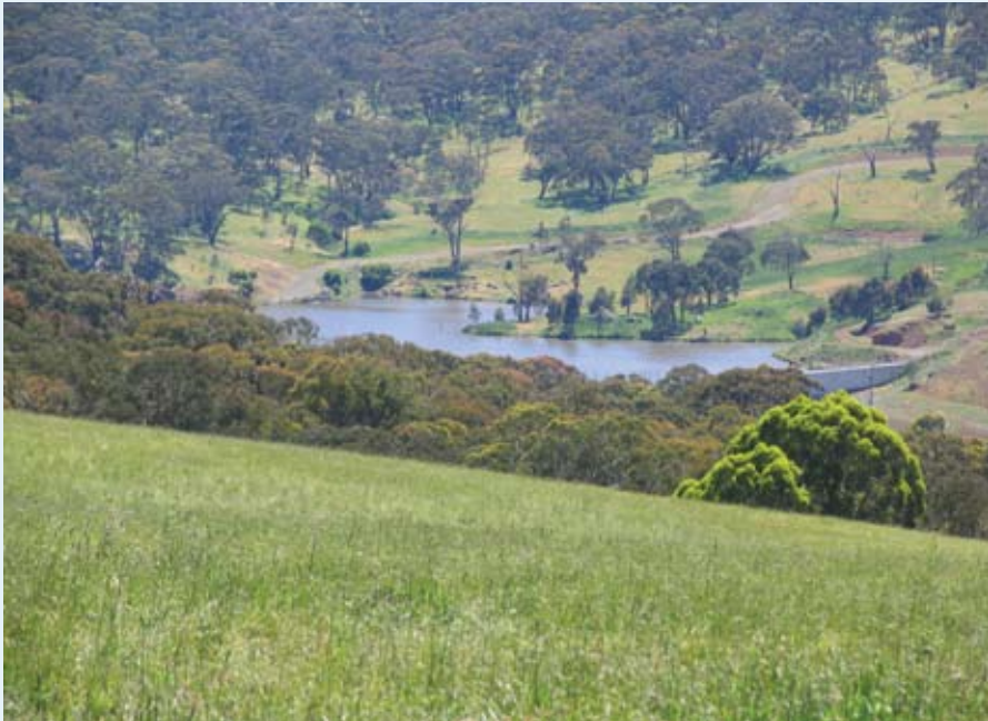
Cadiangullong Creek Dam. Image Source: David Parry, Charles Sturt University
