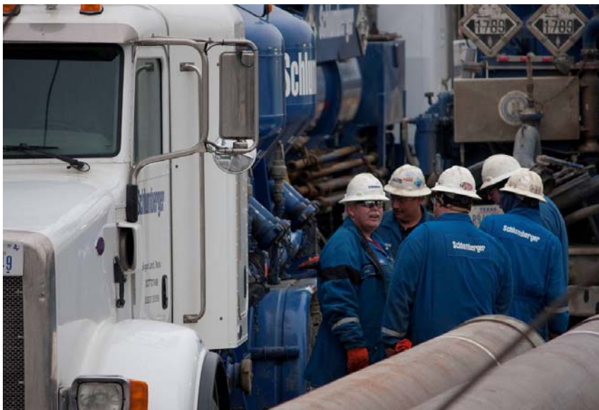
Figure 1 Cementing the surface casing at the Decatur Project, Illinois, USA.
