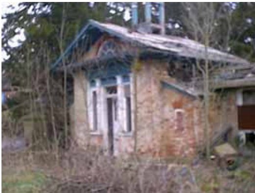
Figure. 40 The dilapidated lodge to Brasted Place
