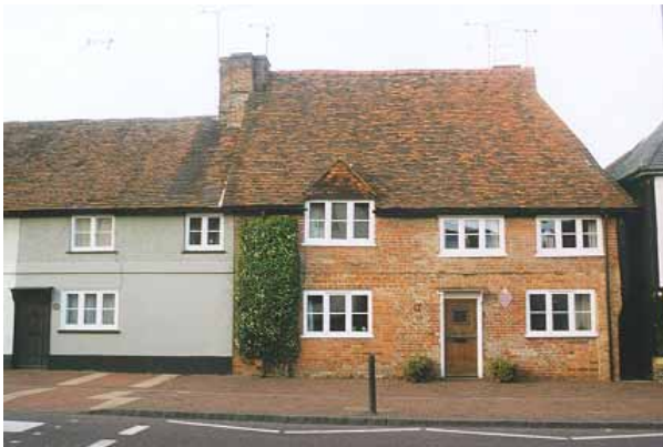
Figure 7 Varying roof lines
