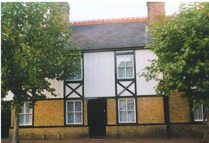
Figure 16 Herringbone patterned brickwork
