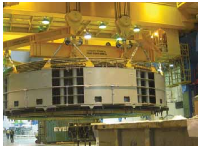
Above: GMS Stator Replacement
