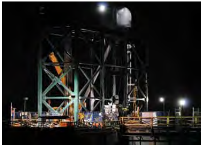
Left: Vancouver Island’s Strathcona Dam at night, as seen by the construction crew who worked 24/7 for five months to ensure the intake tower received necessary seismic upgrades.
