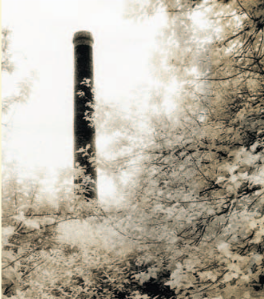
Chimney to the west of the Vivian Engine House
