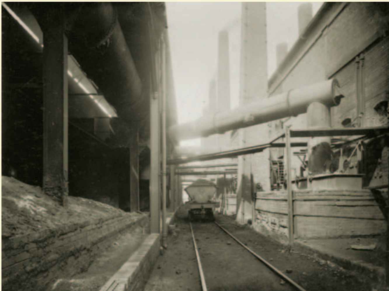
Hafod Copperworks view through works interior
