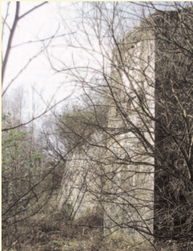
The Copper Slag Abutment
