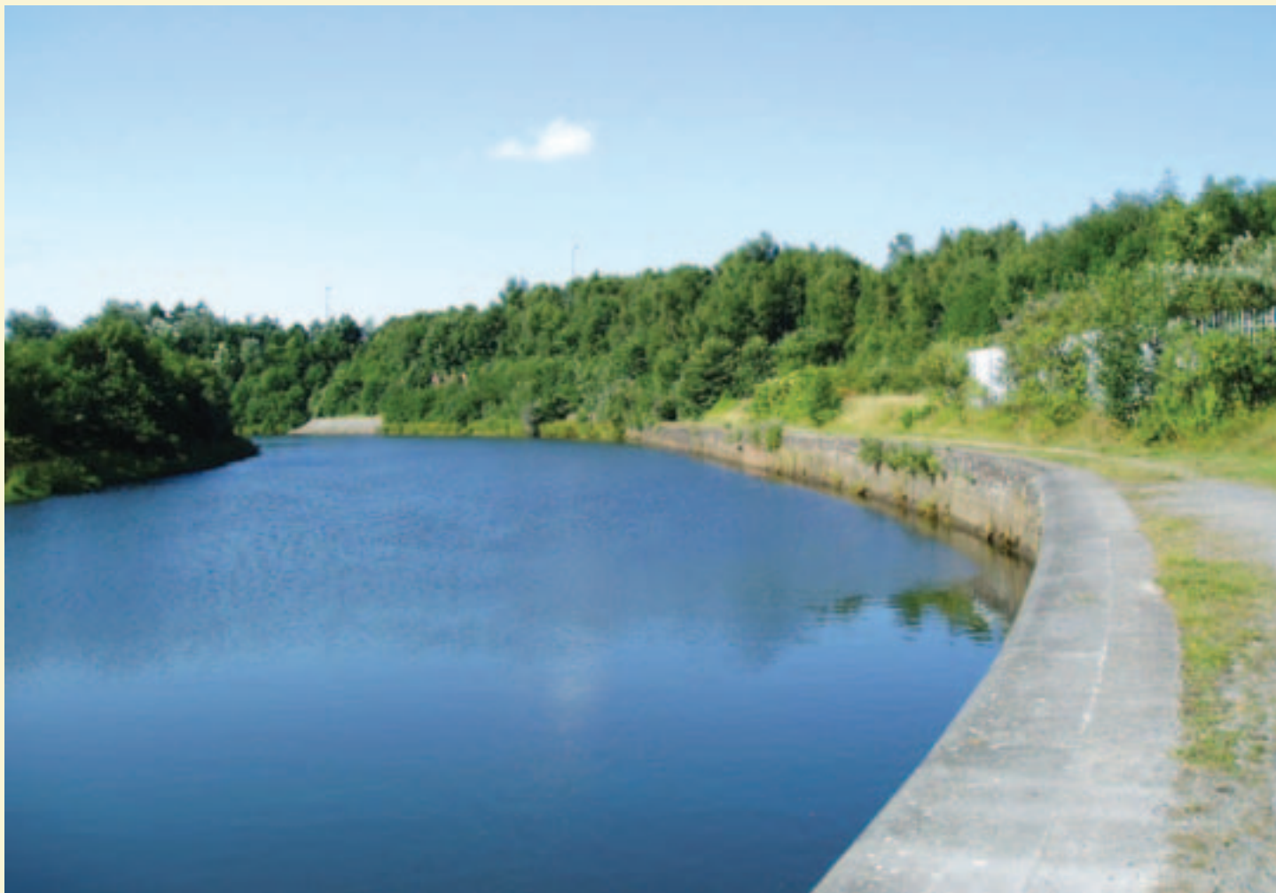
The Hafod Copperworks river quay looking south towards the city centre
