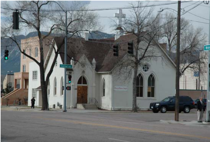
Methodist Episcopal Church / Rose of Sharon Temple 229 East Cucharras Street 1884 / Architect unknown Loop A No. 5
