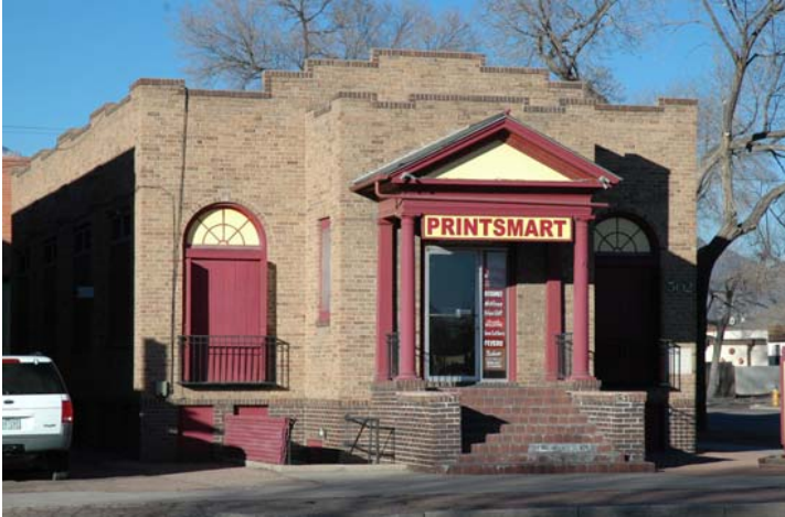
Verner Z. Reed Memorial Library 502 South Tejon Street 1926 / Architect Thomas Hetherington Loop B No. 15
