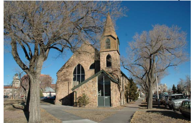
Payne Chapel A.M.E. Church 320 South Weber Street / 128 Pueblo Avenue 1897 / Architect M. M. Ritter Loop A No. 8
