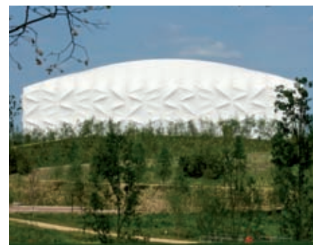
PVC containing phthalate plasticisers used on the Basketball Arena, as the material was procured before issuing the PVC Policy
