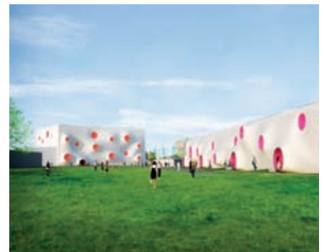
Phthalate-free PVC was used on the temporary shooting ranges at the London 2012 Shooting Venue
