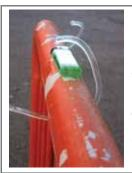
January 2007. This photograph shows an icicle on the railing outside the Annagh Medical Centre, Doctor's Road, in January 2007. What appears to have happened is that water inside the railing froze, expanded and was pushed outwards through a small circular hole in the metal. As it did, the colder temperature outside froze it further it kept expanding, causing the icicle, which eventually curved nearly all the way around the railing! Cigarette lighter shown for scale.
