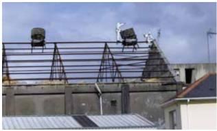
These images were taken in the spring of 2008 when workmen attached to harnesses and wearing protective masks and white body suits began dismantling the old asbestos roof. It took many weeks to complete this part of the project. The first image was taken on 27th March and the second image was taken on 8th April.
